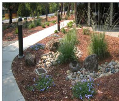
Swales and dry creeks are narrow, linear depressions designed to capture and convey water. Swales imitate a natural creek's ability to slow, infiltrate, and filter stormwater. To install a swale follow these steps:
