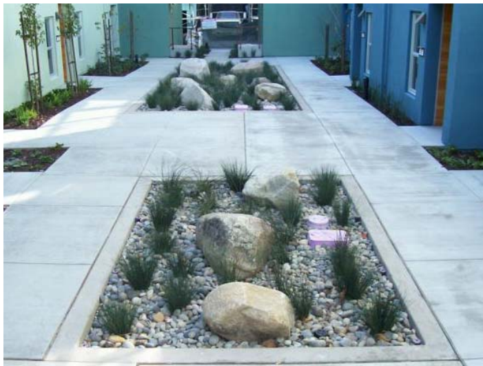
Figure 8-2: Flow-through planter in the City of Emeryville
