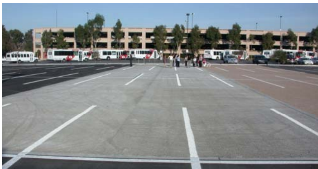
Fig. 8-6 Porous asphalt, pervious concrete and pervious interlocking concrete pavers at Stanford University demonstration project.
