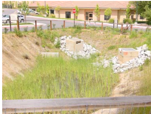
Figure 8-5: Detention pond at a retirement center in Saratoga
